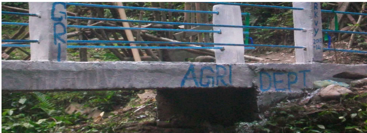
Foot bridge constructed under RKVY 2013-2014
